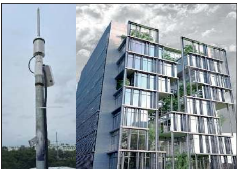
Low Voltage System with Early streamer emission Citizen Tower at Bir Uttam Mir Shawkat Sarak
