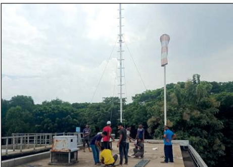
LPS, OPR-60 Saidaabad Water Treatment Plant
