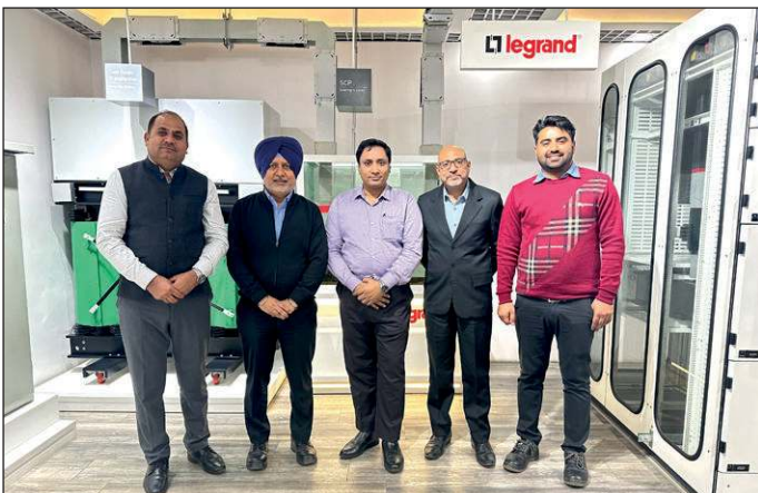
Legrand Delhi, Switchgear Factory Visit 2022
