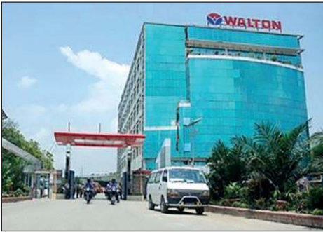
LV Equipment & Measuring Instrument Walton Group
