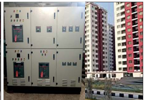
Low Voltage Switchgear Rajuk Utara Apartment Project - RUAP
