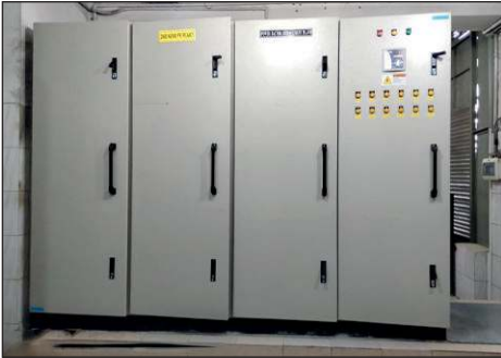
2400 KVAR APFC Grameenphone Switch at Nobinogor, Savar
